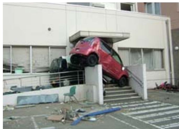
Figure 2. Backdoor of the Onigawa municipal hospital.
